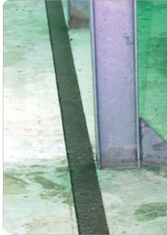
Figure 8 – Laying the bituminous strips
