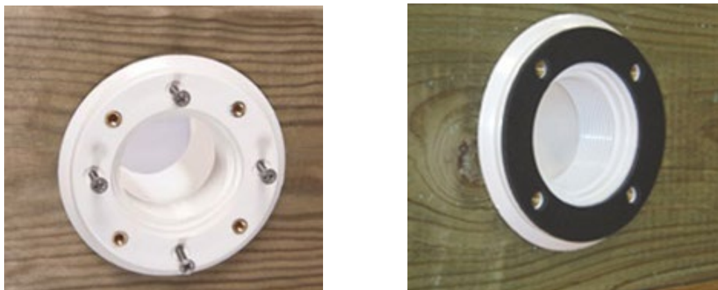
Figure 24 – Mounting the return fitting body and gasket
